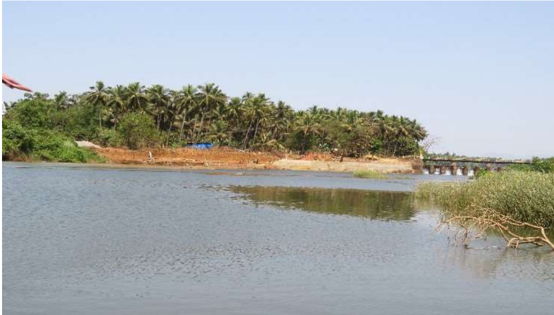
Figure 9.5: Constriction of protective wall/embankment opposite Sal water treatment plant.
